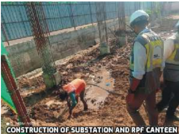
CONSTRUCTION OF SUBSTATION AND RPF CANTEEN stage-I.
